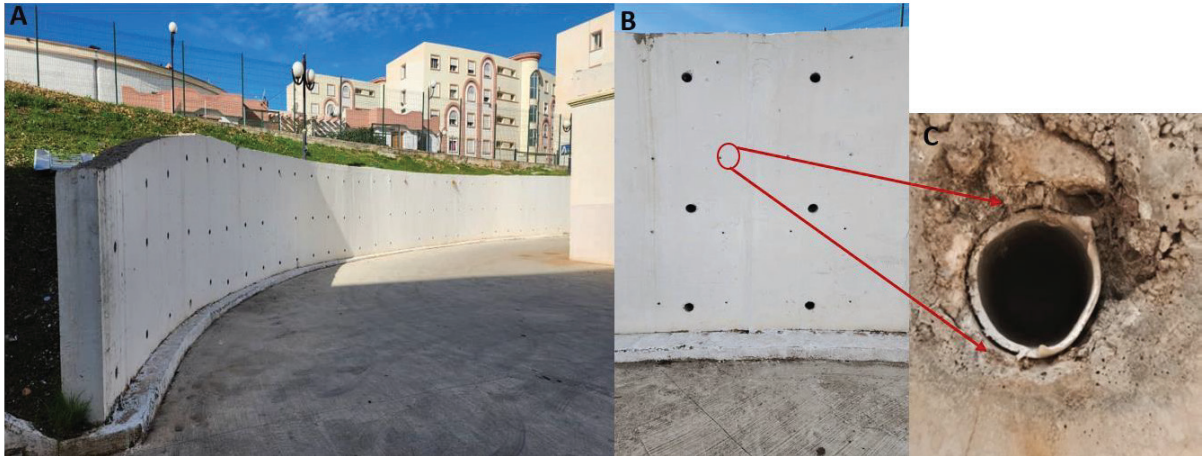
Figure 3. A) An overview of the concrete wall; B) Tie holes on the wall; C) Enlarged photo of a tie hole.
